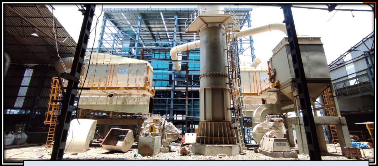
Sand plant, Shake out Sand Cooler DES Erection done
