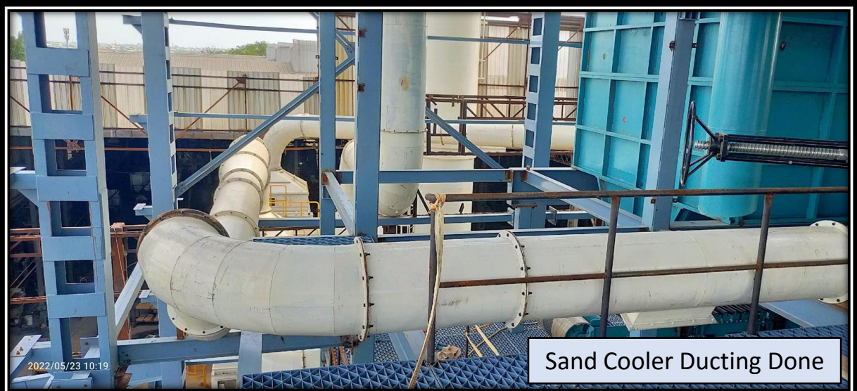
Sand plant, Shake out Sand Cooler DES Erection done
