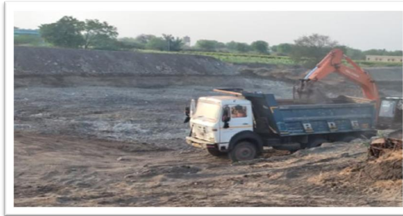
Removing of weeds & Silt
