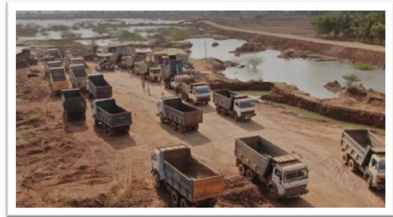
Heavy Machineries & Equipment Mobilization
