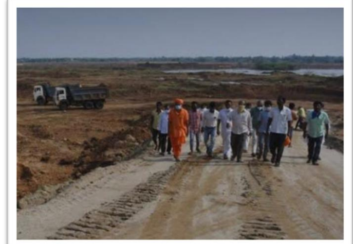
Approach Road Preparation Review
