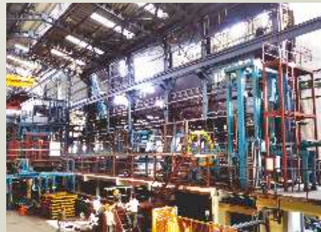
Moulding Line Under Installation at Koppal
